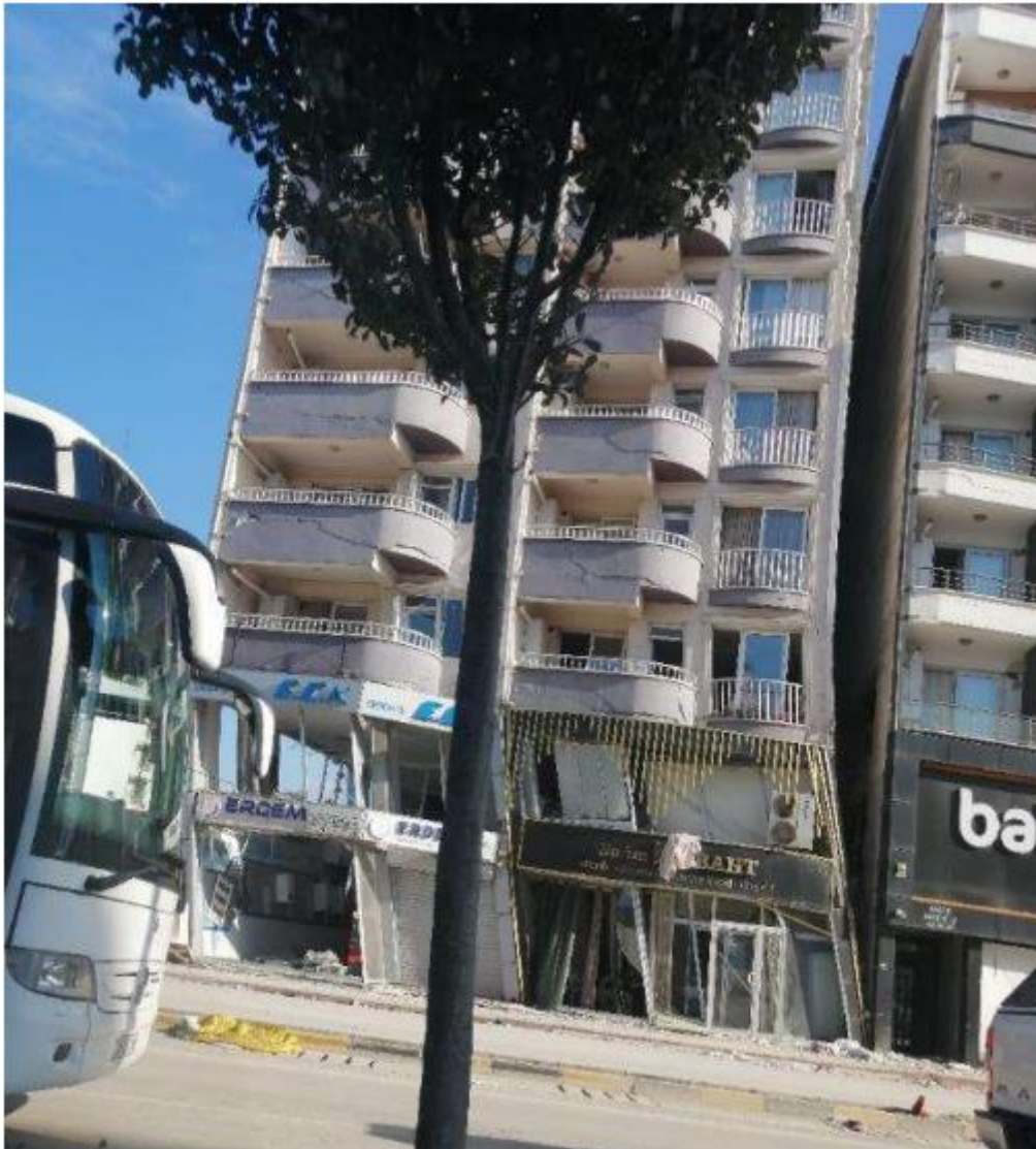
Figure 4 Soft Storey Example
