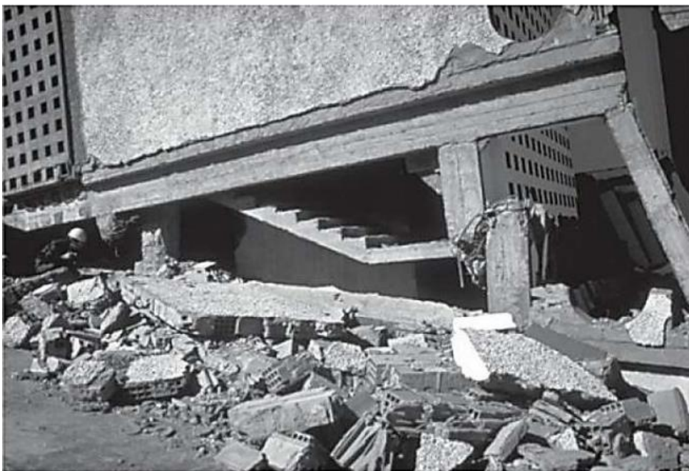
Figure 5 Short Column Effect Example
